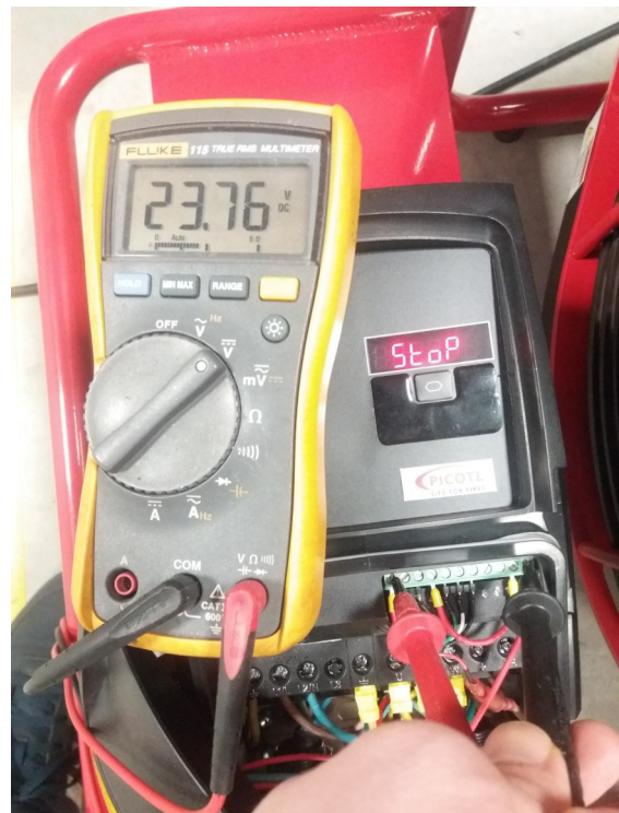
Emergency stop pressed
